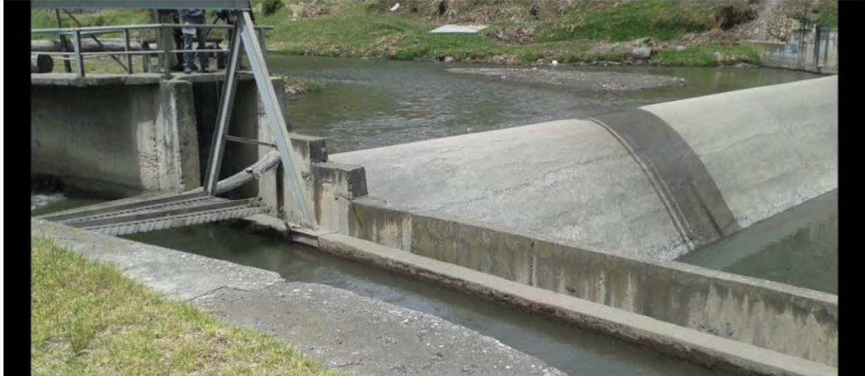
Figure 17: Example of a lateral water intake behind a diversion weir.
