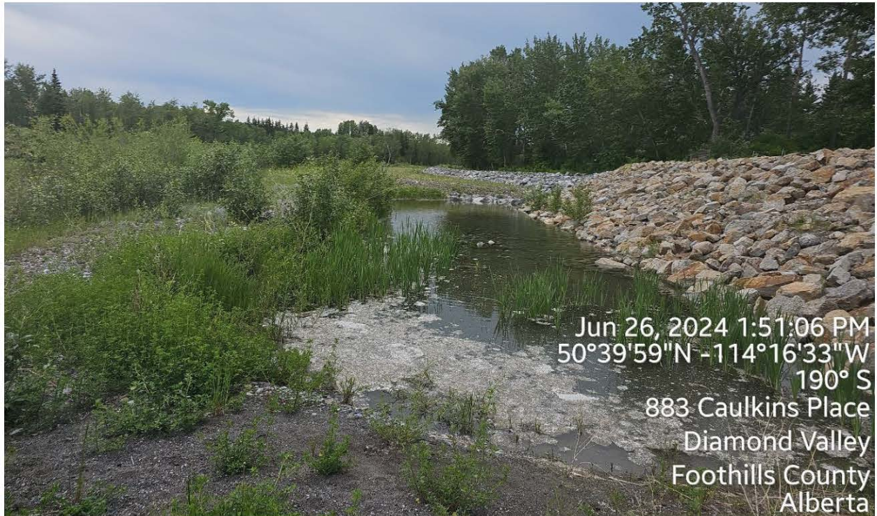
Figure C-3: Flood protection berm at the left side of the Sheep River floodplain.
